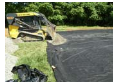
Adding Gravel onto Filter Cloth
