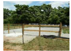
Finished Heavy Use Area
