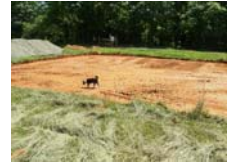
Grading for Heavy Use Area
