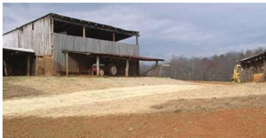
This steep hillside was eroding and delivering sediment to a nearby stream. Intensive grading and shaping was completed prior to seeding according to NRCS specifications. A diversion was constructed to divert water to an established vegetated outlet. One of the keys to a successful stand of grass is the proper spreading of a protective cover ■
